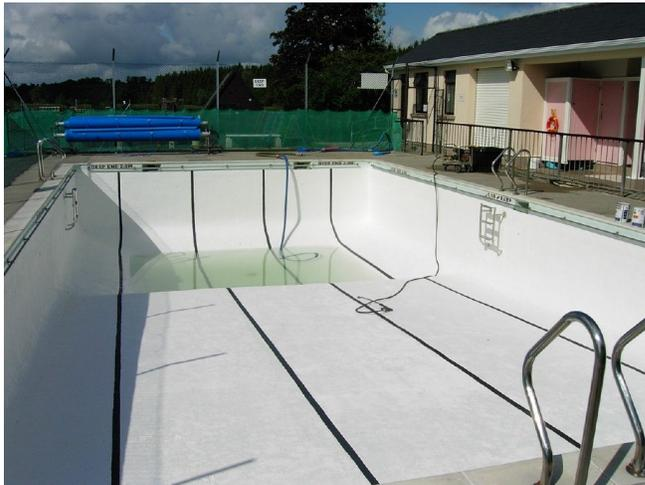
In this case, **Fortachlor Q800 Chlorinated Rubber Swimming Pool Paint** has been applied to the floor and walls of an outdoor pool. Most paints will not stand constant immersion in water, but **Fortachlor Q800 Swimming Pool Paint**, when the surface has been properly prepared, and the conditions right during application, will give a long life protective finish.
